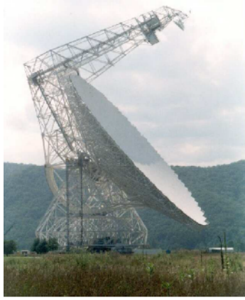
(a) The 110\text{m} \times 100\text{m} diameter Green Bank Telescope is the largest steerable radio telescope. It has an off-set feed and unblocked aperture, giving an aperture efficiency of 0.71 at longer wavelengths.
