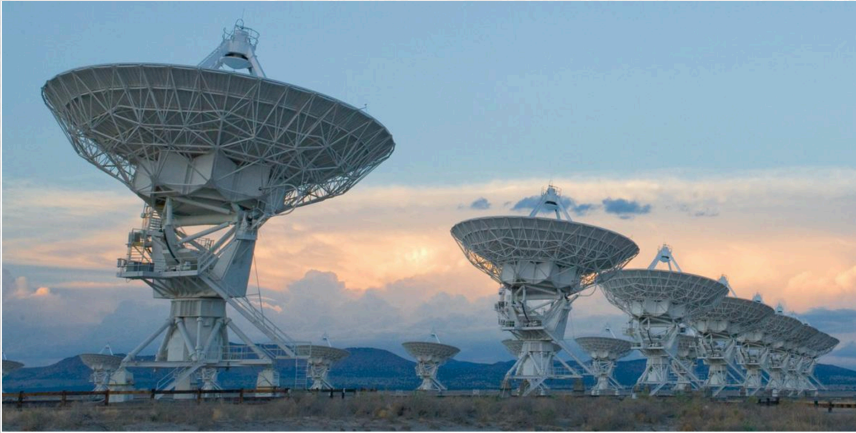
The Very Large Array (VLA) is a collection of 27 radio antennas located at the NRAO site in Socorro, New Mexico. Each antenna in the array measures 25 meters (82 feet) in diameter and weighs about 230 tons. Credit: Alex Savello/NRAO
