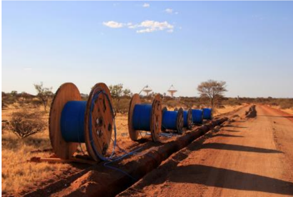
Installation of optic fibre during construction of the ASKAP antennas and associated infrastructure in 2011.
