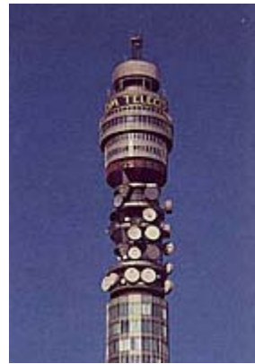
Figure 2.5: The Post Office Tower in London is the heart of the UK network of microwave telecom links. Older readers may remember that originally the antennas on the tower were smaller versions of the Bell Labs horn.
