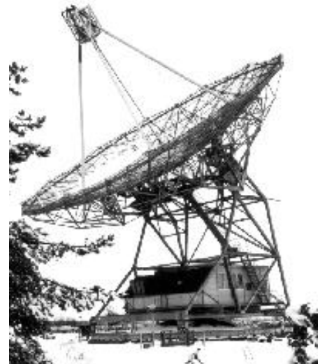
Figure 17. The 25-metre Dutch antenna at Dwingeloo - one of the earliest large fully-steerable parabolic telescopes.
