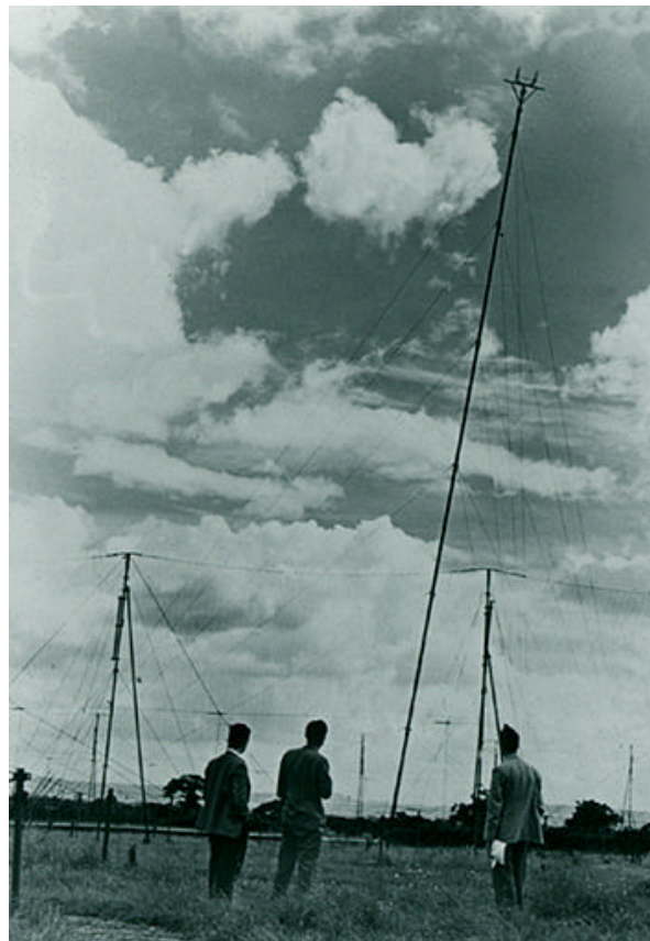
Figure 11. The 218ft antenna at Jodrell Bank which detected radio emission from M31, the nearby large spiral galaxy in Andromeda.
